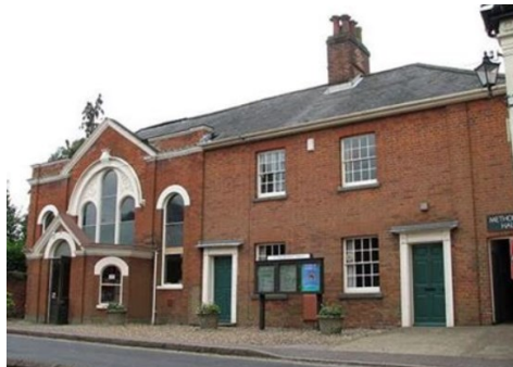
Aylsham Methodist Church
